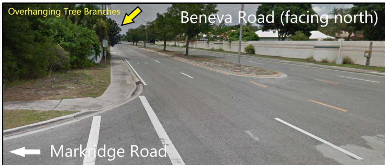
Figure 11 – Overhanging Tree Branches
